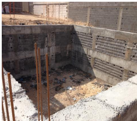
(A) Septic Tank Wall
